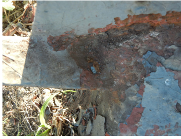
(a) Image taken close to the structure
